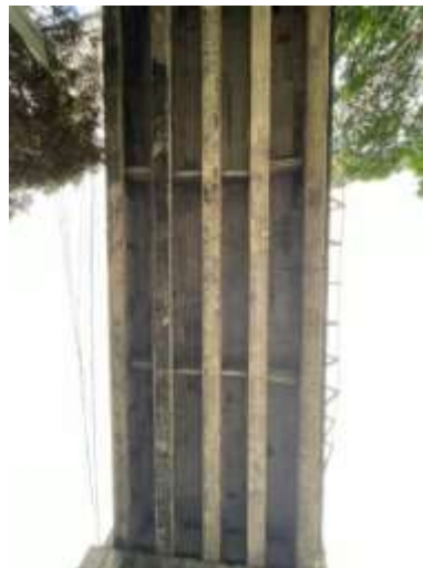
Figure 9. Application of Prestressed Technology and Pile Foundations
