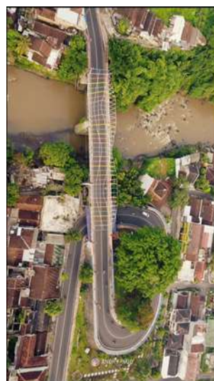
Figure 5. The Trumpet Interchange Configuration of the Semanggi Bridge in Jember
