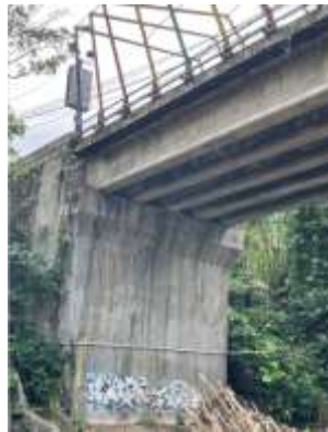
Figure 6. Structural Components of the Semanggi Bridge, Jember.
